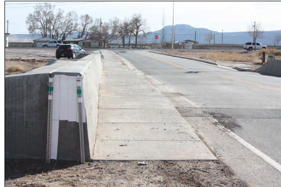
Figure 13. Terminating Sidewalk Example
